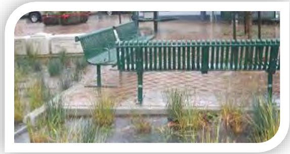
Green stormwater infrastructure is designed to mimic natural processes. This photo shows how landscaped bioretention areas help to detain and slow the flow of stormwater runoff to the storm drain system (Source: Nevue Ngan).
