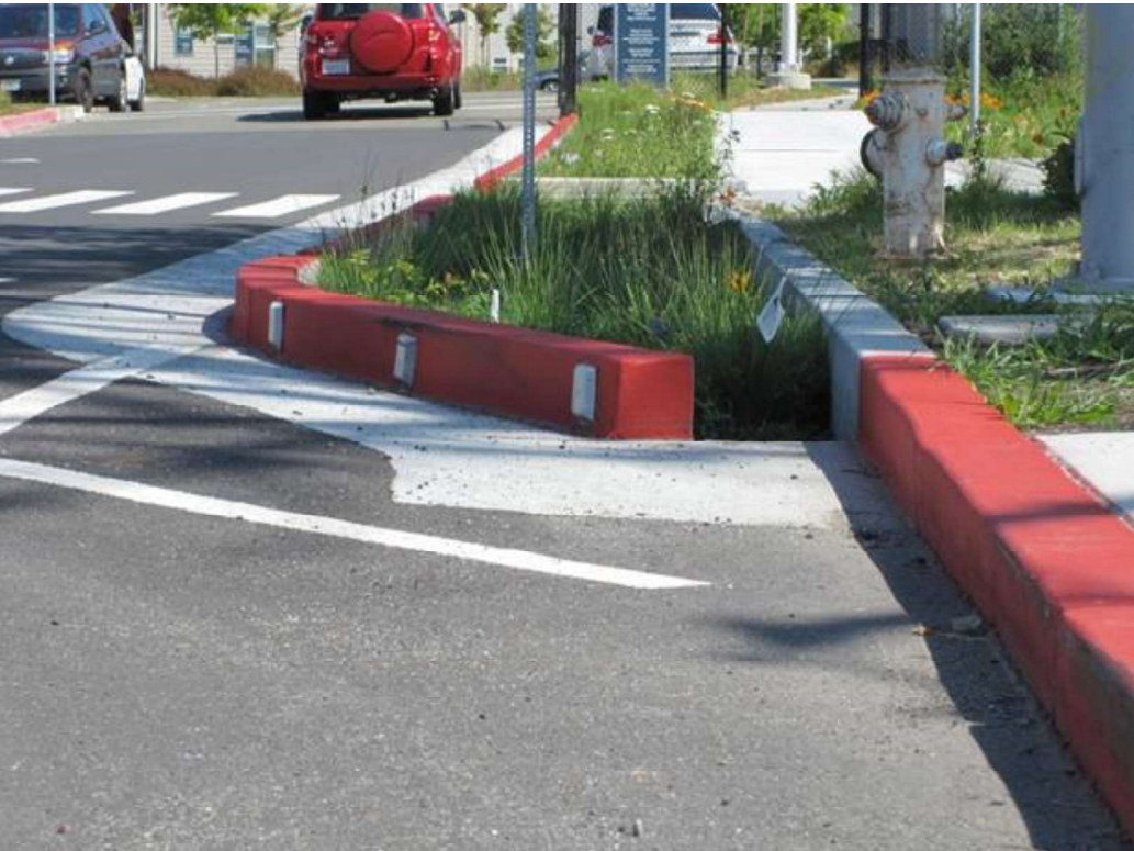
Figure 2: In-line system in Berkeley/Albany where low and high flows enter the system and overflows exit through a drain within the system.
