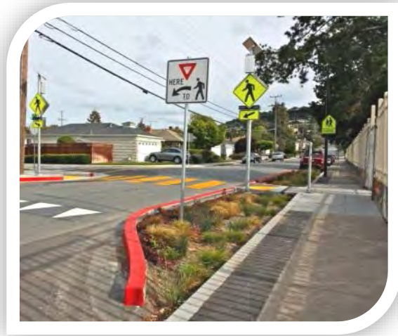
Sustainable Street in the City of San Mateo; stormwater runoff flows into a “bioretention area” or rain garden that reduces the crossing length for pedestrians near a local school (Source: SMCWPPP).
