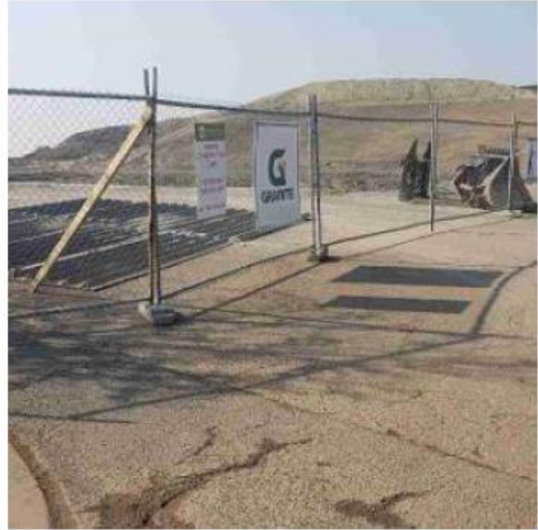
Exits have been swept and cleaned. No sediment track out is present.
