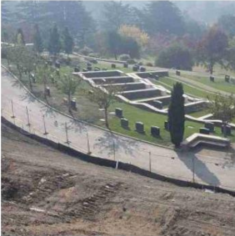
Silt fence has been repaired at base of slope.
