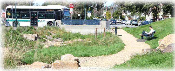
Bioretention facility in El Cerrito with active and passive recreational uses.
