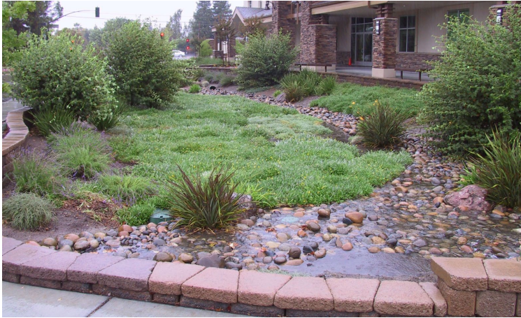
Bioretention facilities can be rectangular, linear, or nearly any shape. Photo by Scott Wikstrom
