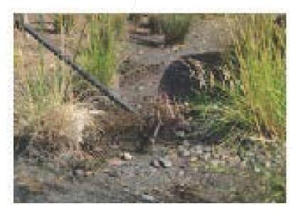
Sediment removal should occur during the dry season. If sediment is wet it needs to be dewatered before disposal. Do not drain wet sediment outside the facility (pollutants will enter the SD!)
