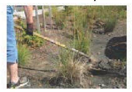
Put sediment in a bucket/wheel barrow and dispose in regular trash (not yard waste)
