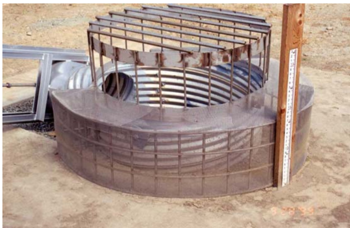
Figure 1 Example of Extended Detention Outlet Structure
