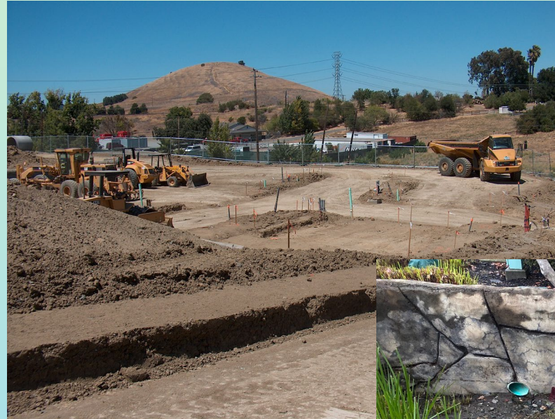
Belmont Terrace under construction – 2008
