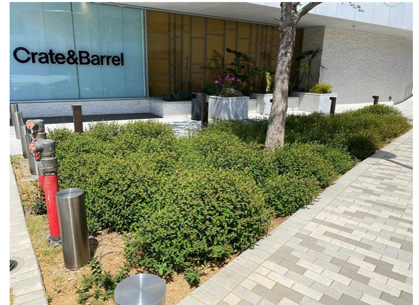
Flow-through Planters at Broadway Plaza in Walnut Creek
