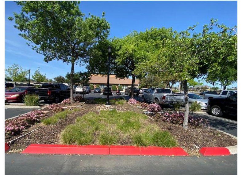
Bioretention at Oakley Civic Center
