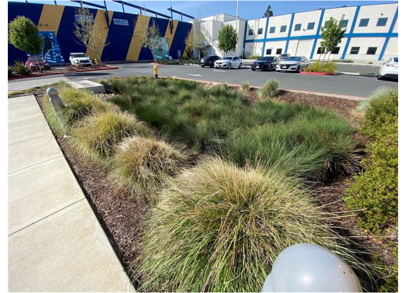
Bioretention at Shadelands Sports Complex in Walnut Creek
