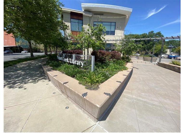
Walnut Creek Public Library Flow-through Planters
