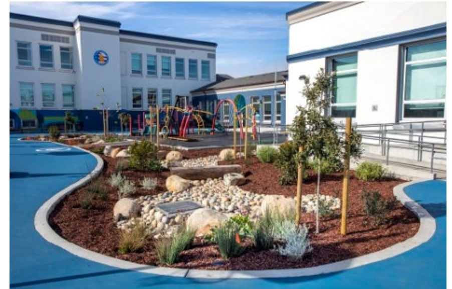
Lafayette Elementary received a stormwater retrofit from San Francisco's Large Green Infrastructure Grant Program
