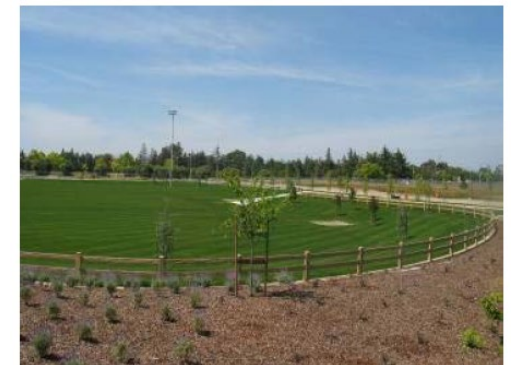
Figure 7-5: Example of a multi-purpose detention facility for HM control in San Jose.
