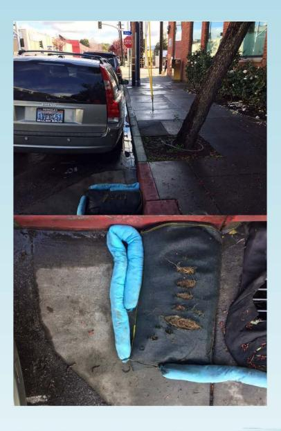
Public Works staff, as mentioned, had placed absorbent socks at intervals along the curb. After the source was cleaned up, the gutter was clear past the first absorbent sock; this photo was taken at around 11:30 near the spot the first photo, above, was taken:
