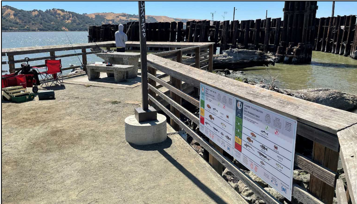
Figure 5. New sign installation at Radke Martinez Regional Shoreline Fishing Pier - overview
