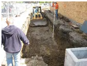
Figure 4-2. Excavation of IMP #2 at Pittsburg Site.
