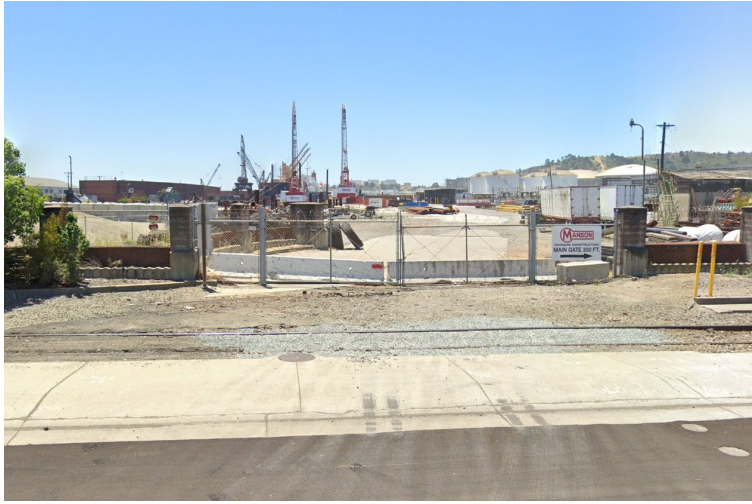
Parcel #4 (view along Cutting Blvd)
