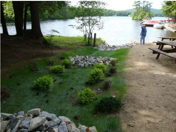
Figure D-35 Examples of Vegetated Swales
