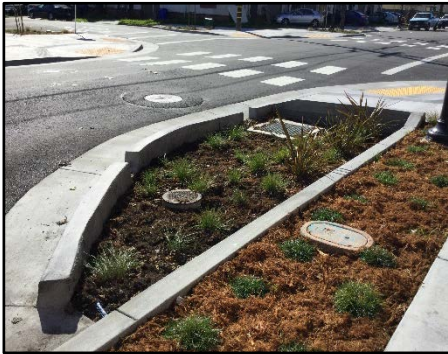
Figure D-39 Bioretention Profile Schematic and Examples
