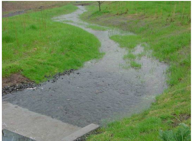
Figure D-35 Examples of Vegetated Swales
