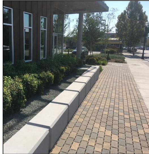
Pervious Pavement in Walnut Creek (Pervious Asphalt Left and Pervious Pavers Right) are Examples of Multi-Benefit Stormwater Projects that Promote Water Infiltration in Areas Where Vegetation is Not Appropriate
