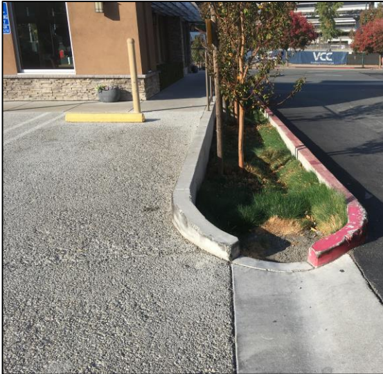
Pervious Pavement in Walnut Creek (Pervious Asphalt Left and Pervious Pavers Right) are Examples of Multi-Benefit Stormwater Projects that Promote Water Infiltration in Areas Where Vegetation is Not Appropriate
