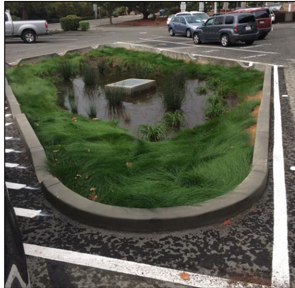
Unlined Bioretention Retrofit in the County Public Works Building Parking Lot
