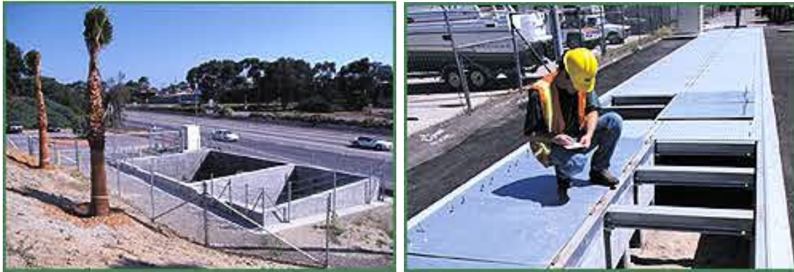
Figure B-8. Caltrans Pilot Media Filters (Austin Sand Filter [left], Delaware Sand Filter [right])
