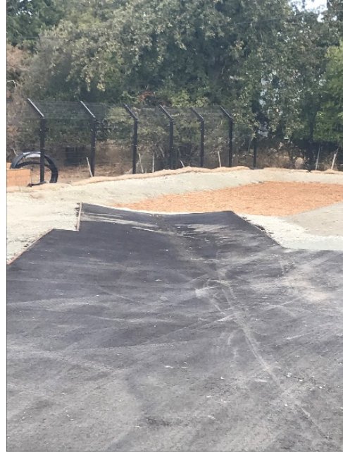
Photograph of new paving and bio-swale
