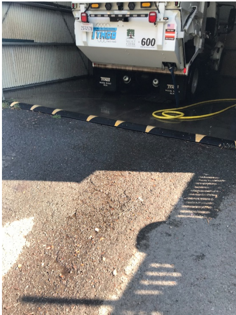
Photograph showing newly installed berm at wash pad.
