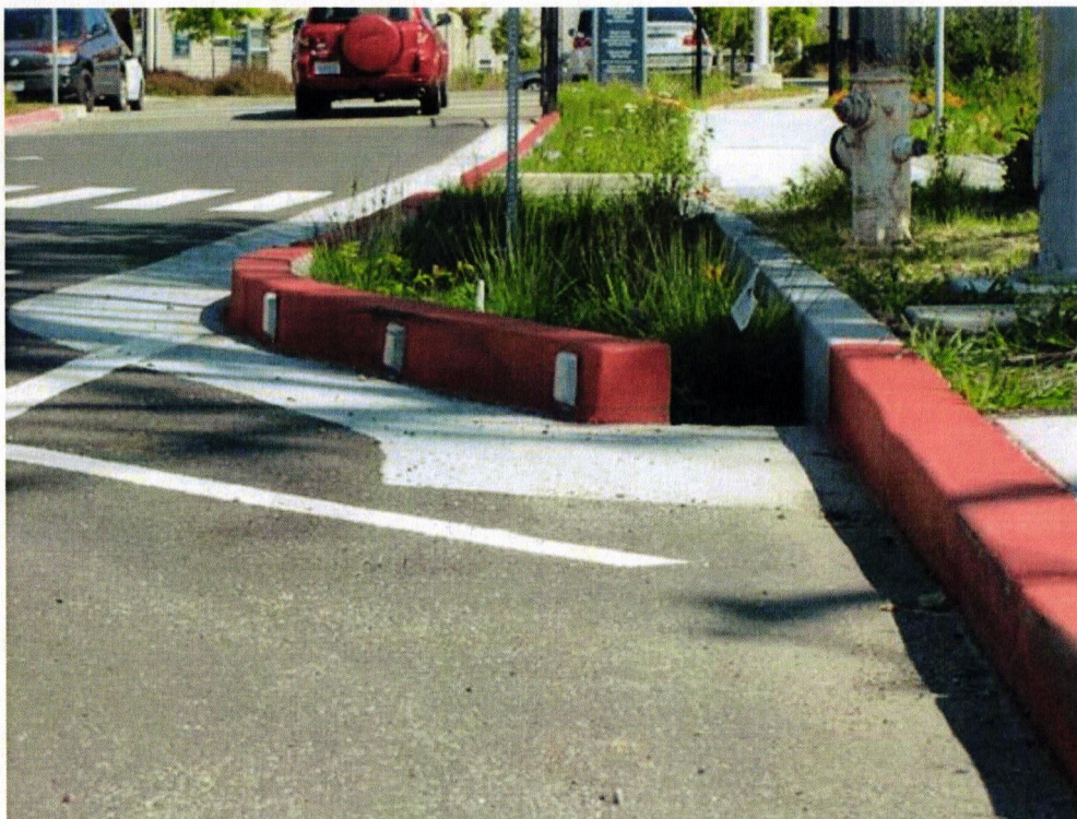
Figure 2: In-line system in Berkeley/Albany where low and high flows enter the system and overflows exit through a drain within the system.
