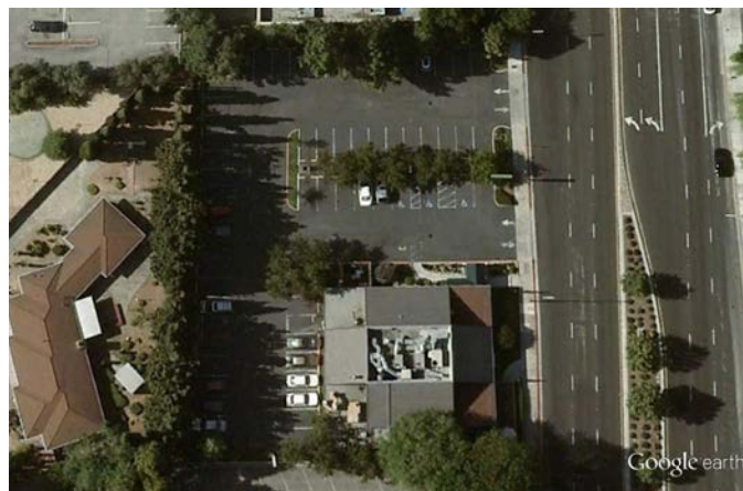
Figure 2. Existing Site Conditions.
