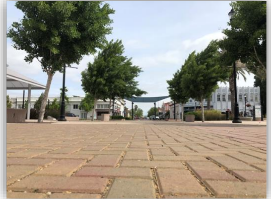
John Buckley Square permeable pavement
