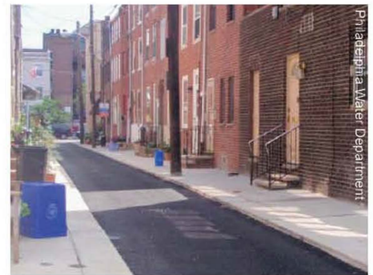
Philadelphia (pervious pavement)
