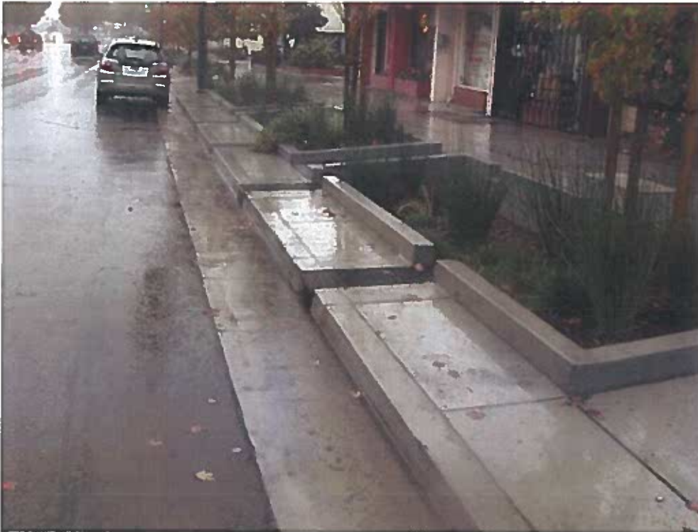
Figure 1: Off-line system in El Cerrito where low flow is diverted to the sidewalk planter and high flows continue down the gutter.
