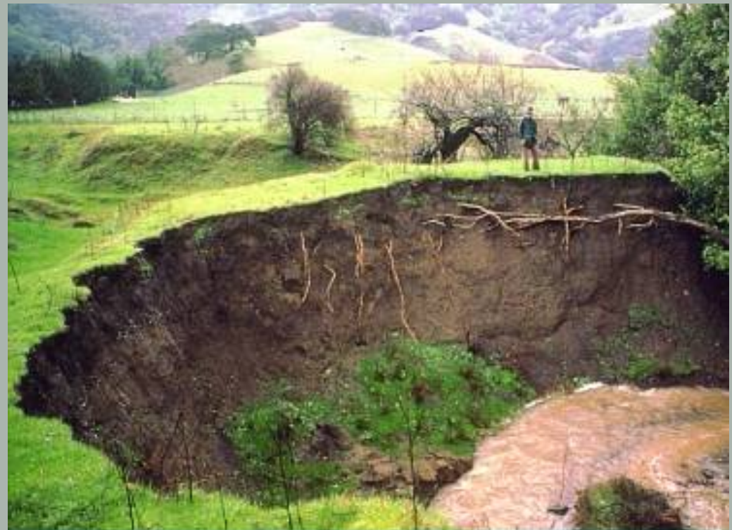
Pre-project erosion along Miller Creek
