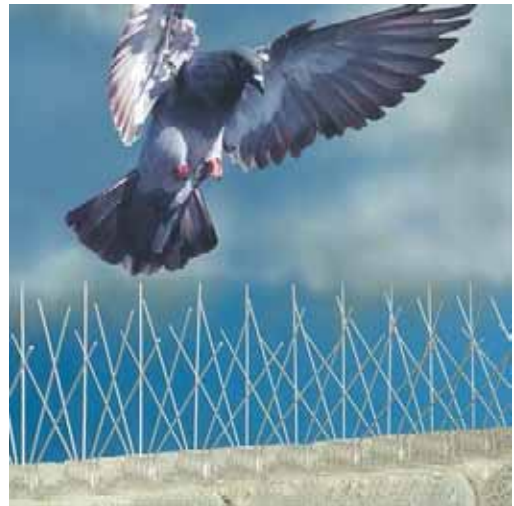
Metal spines installed on a ledge to prevent pigeons from landing or roosting.
