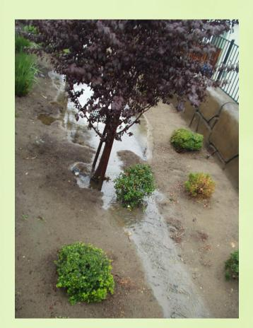
The ponding area should be far larger.  Bioretention Areas should be graded as flat as possible to prevent channelization.
