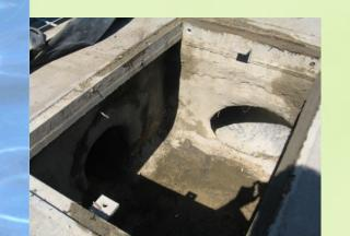
Some initial installations flawed, with the flow line of bypass pipe lower than that of treatment pipe.
