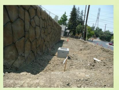
This bioretention area has to be redesigned due to a conflict with an unknown underground pipeline.
