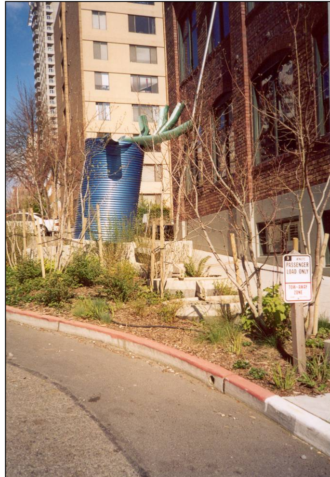
Bio downspout Cistern & Cascade
