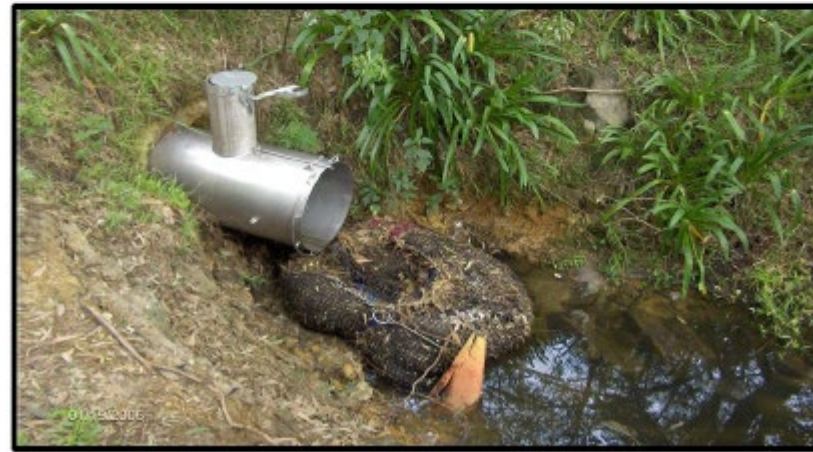
Figure 1. Net filled to capacity and self-detached awaiting routine maintenance.
