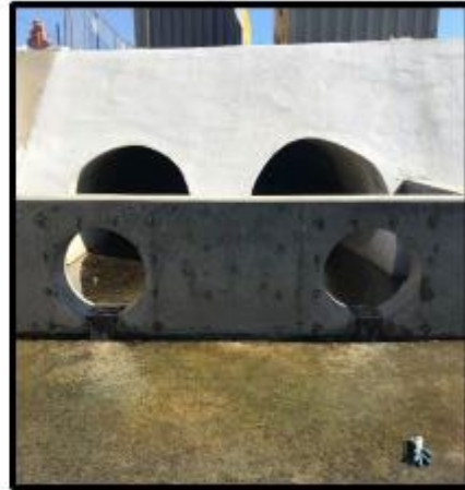
Figure 3. Installed headwalls for mounting NetTech for 100% trash capture of outlet.
