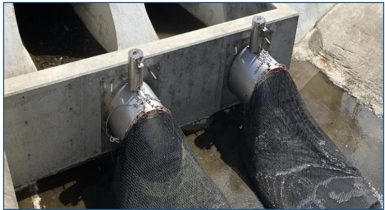
Figure 3.6. NetTech FTC netting system installed in the City of Livermore (Image courtesy of Schaaf and Wheeler Consulting Engineers).
