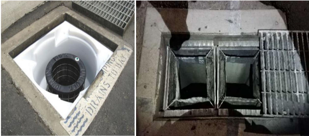
Figure 4.2. (Left) Catch basin insert manufactured by Revel Environmental Manufacturing, Inc. (Right) FloGard® Grate Inlet Basket manufactured by OldCastle (FloGard® GIB) (Images from CASQA https://www.casqa.org/resources/trash/certified-full-capture-system-trash-treatment-control-devices ).
