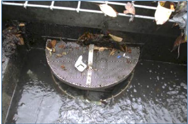
Figure 4.6. Overflowing outflow screen FTC device due to a clogged/occluded screen. Courtesy of SCVURPPP and SMCWPPP (EOA 2016).
