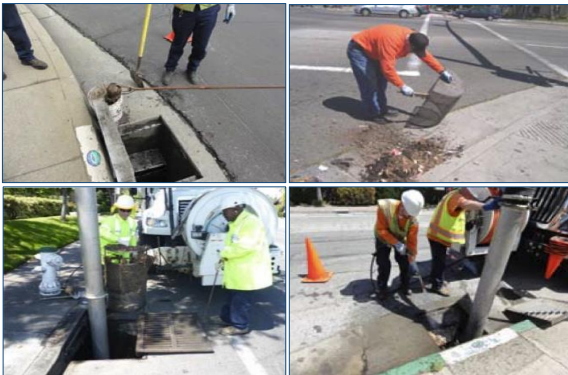
Figure 4.3. Small-scale FTC device maintenance, (Top) manual cleaning and (Bottom) cleaning process by using a vacuum-assisted truck (Photos courtesy of SCVURPPP and SMCWPPP (Image courtesy of EOA, Inc).
