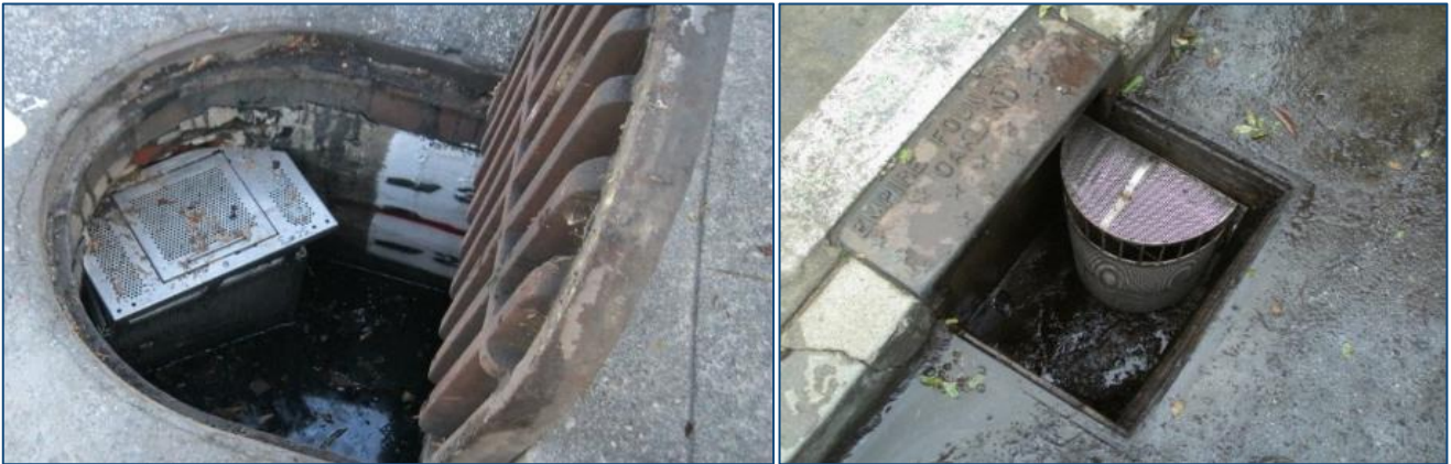
Figure 4.1. Outflow screens installed in catch basins within the Bay Area (Image courtesy of EOA, Inc.).
