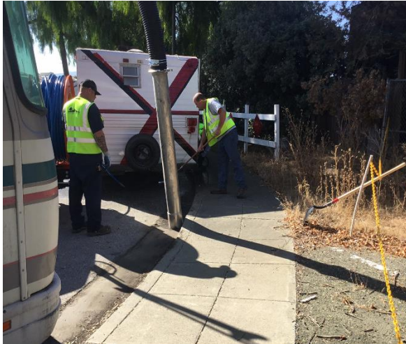
Staff using a vacuum truck to clean an illicit RV discharge. Image courtesy of City of Mountain View.
