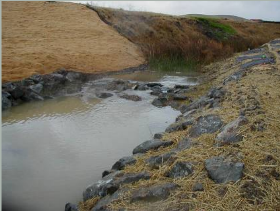
Immediately after installation
