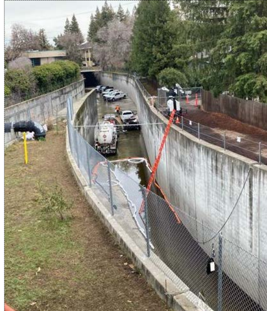
Figure 2, 3. Flood Control Channel clean-up efforts (vac trucks, absorbent booms and pads.)
