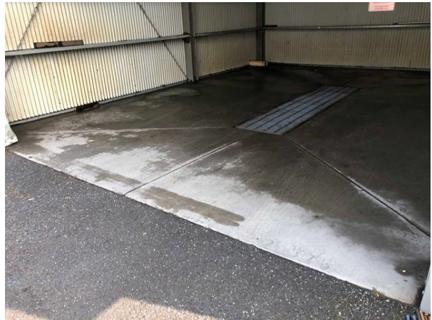
Heather Farm Corp Yard wash pad entrance, before and after, berm installation (2020).
