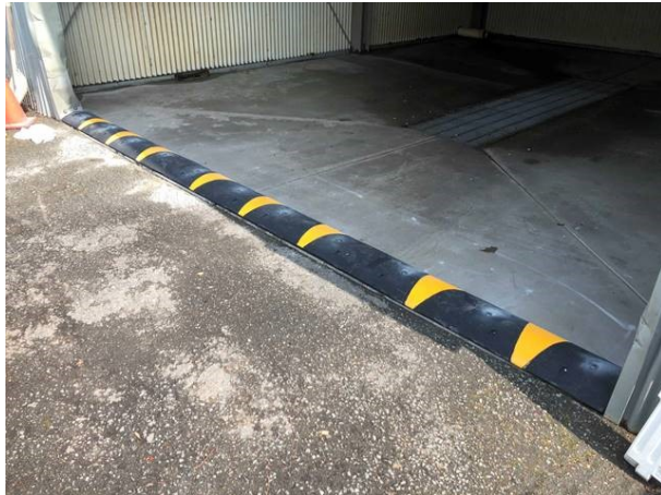
Heather Farm Corp Yard wash pad entrance, before and after, berm installation (2020).
