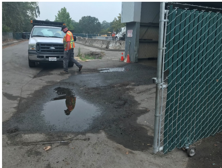
Photograph showing pooled water outside wash pad.
