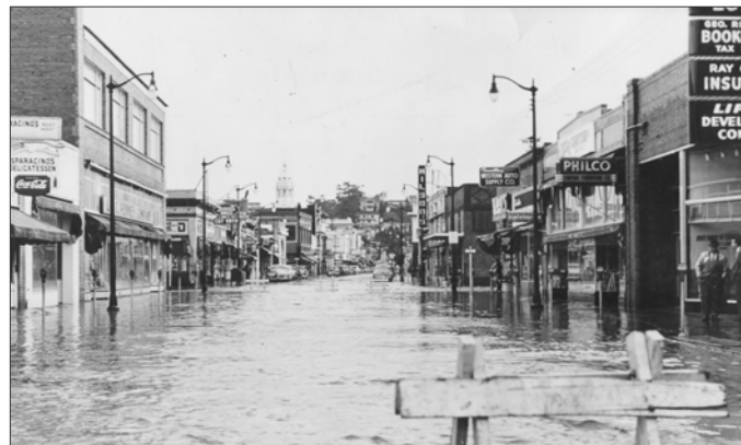
Alhambra Creek floods downtown Martinez, 1955
